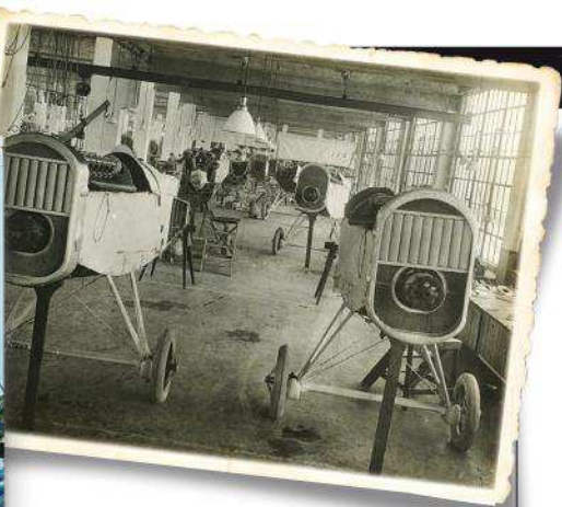
LIBERTY BOMBERS DH-4 fuselages with Liberty engines are assembled at the Dayton-Wright Company factory.
